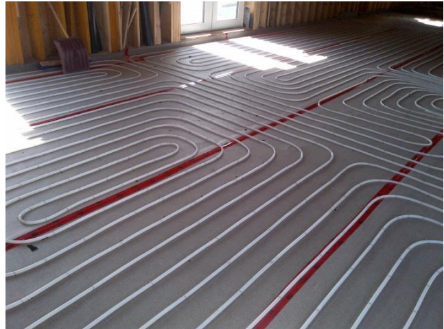
Figure 4 – Installation of In-Floor heating and Cooling at Q Lofts (Polycorp, 2013)
