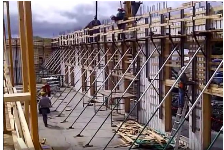
Figure 1 – ICF Construction at Q Lofts (Polycorp, 2013)
